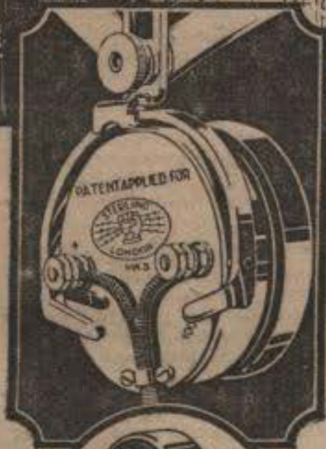
The swivel and trunnion movement and adjustable thumbscrew.
